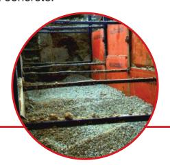
The upper edges of the panels are very robust and the rails have been equipped with integrated protective rails. This means that even difficult jobs will not necessarily be followed by high repair costs. ALLROUND box systems are compatible with sliding trench lining.
